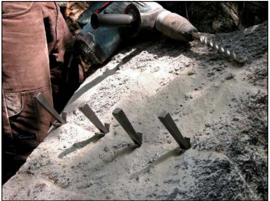
After rifting your rock, holes are drilled at the same angle as the rocks natural resting place. After drilling, feathers and wedges are hammered in at equal intervals, eventually splitting the rock along the rifted seam.
